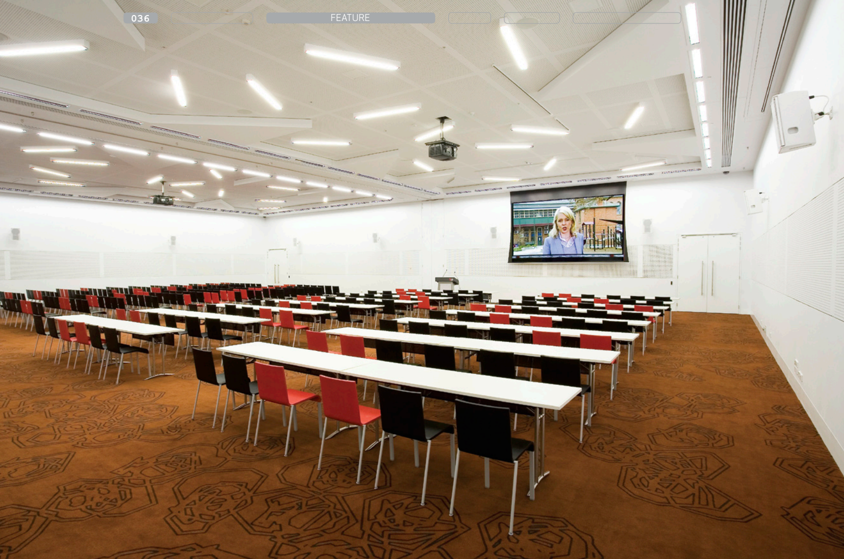
Above: two rectangular meeting rooms joined together. The duplicated sets of speakers for long mode and wide mode can be seen in each room. The retracted wide mode screen for the right hand room is also visible. Note also the diagonally oriented fluorescent light fixtures. Right Top: a standard MCEC lectern with its dual touch screens, gooseneck mics, cough button, direct USB socket and discreet LED document lighting. Right Bottom: meeting room racks in a local control room
